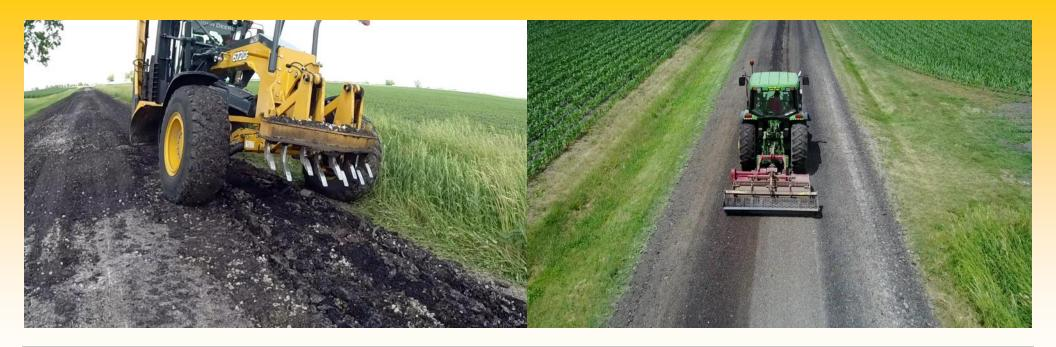
For tractor's not equipped with a Creeper Gear, it's necessary to Scarify/Rip before using Road Grinder
